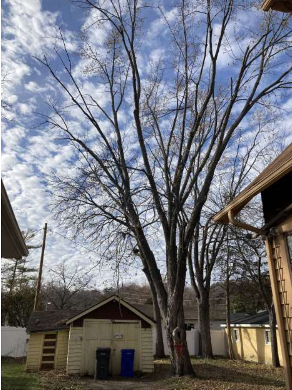
955 May St.Dangerous Tree Photos
